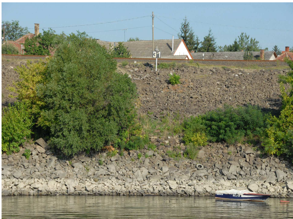
Figure 25: Rip-rap embankment at rkm 1,531
