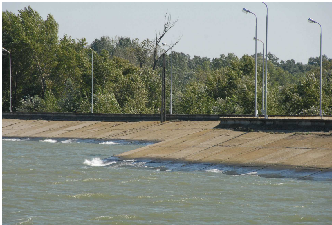
Figure 30: Concrete bank within Iron Gate II at rkm 866
