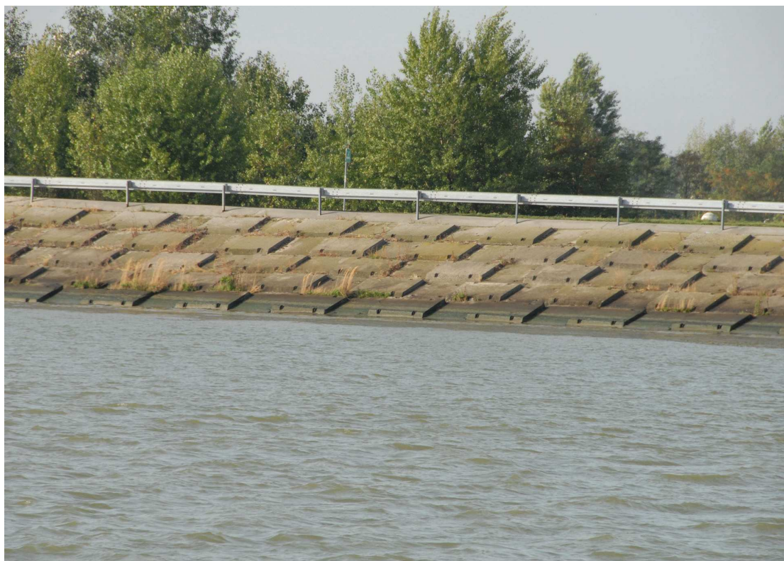
Figure 17: Concrete bank reinforcement at rkm 1,852
