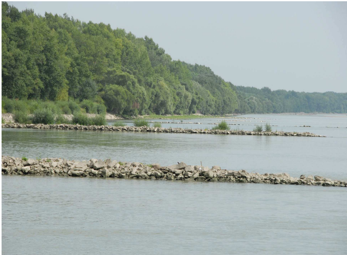
Figure 18: Groyne fields mostly as low water regulation for navigation at rkm 1,805
